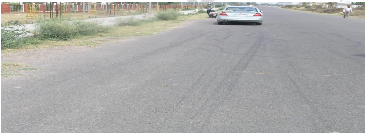
Fig-2: Showing Skid Marks Left by a High Speed Vehicle
